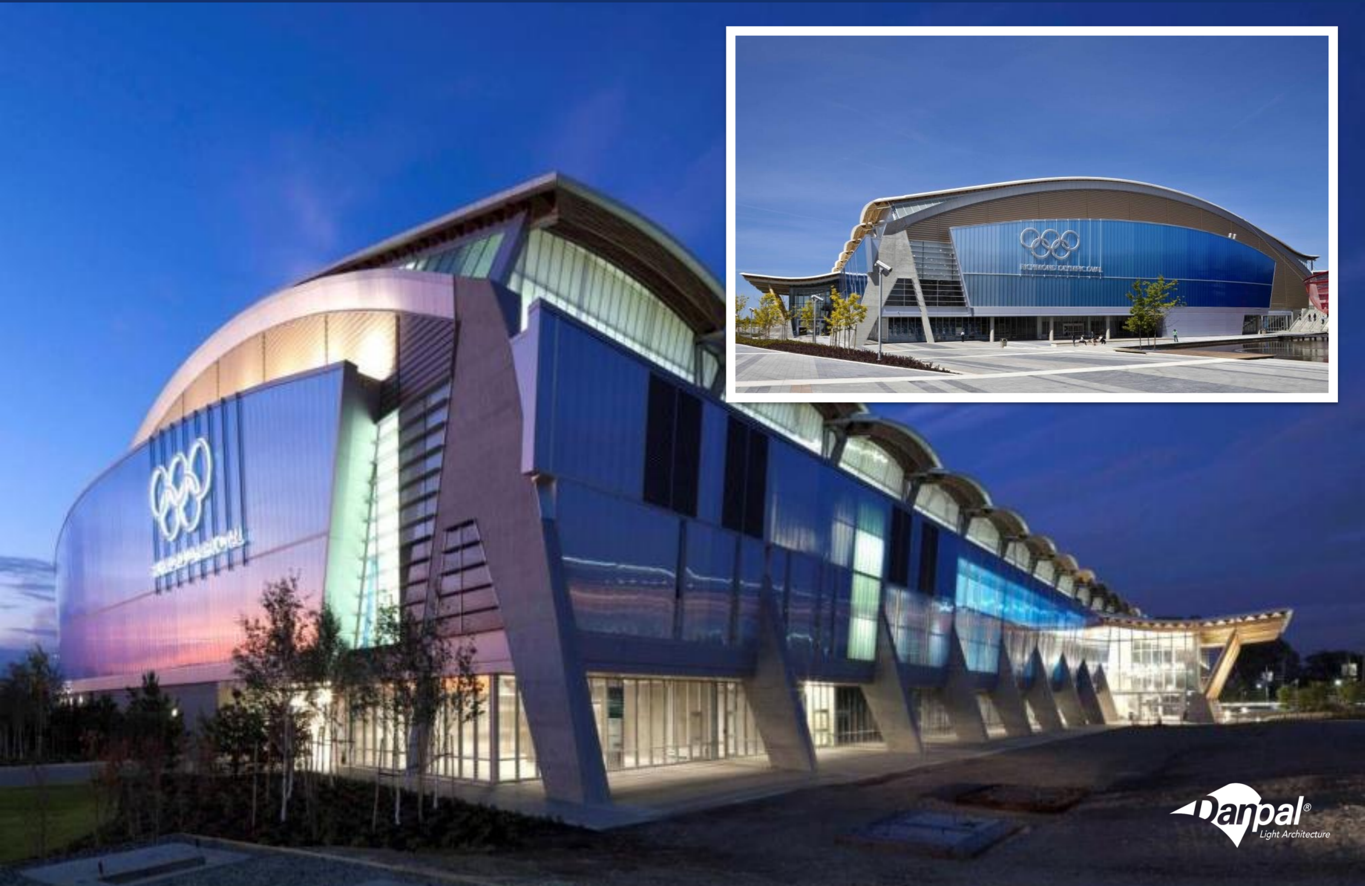
Swimming-Pool, CPI daylighting ing, Canada
