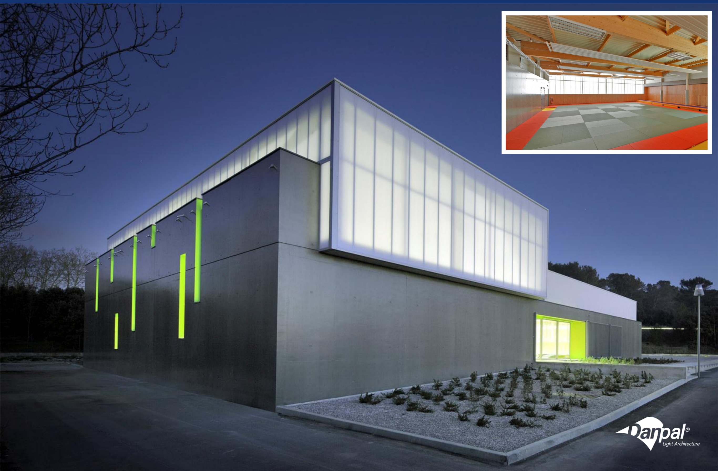
Gymnasium, Architect: Matte Devaux Rousseau, France
