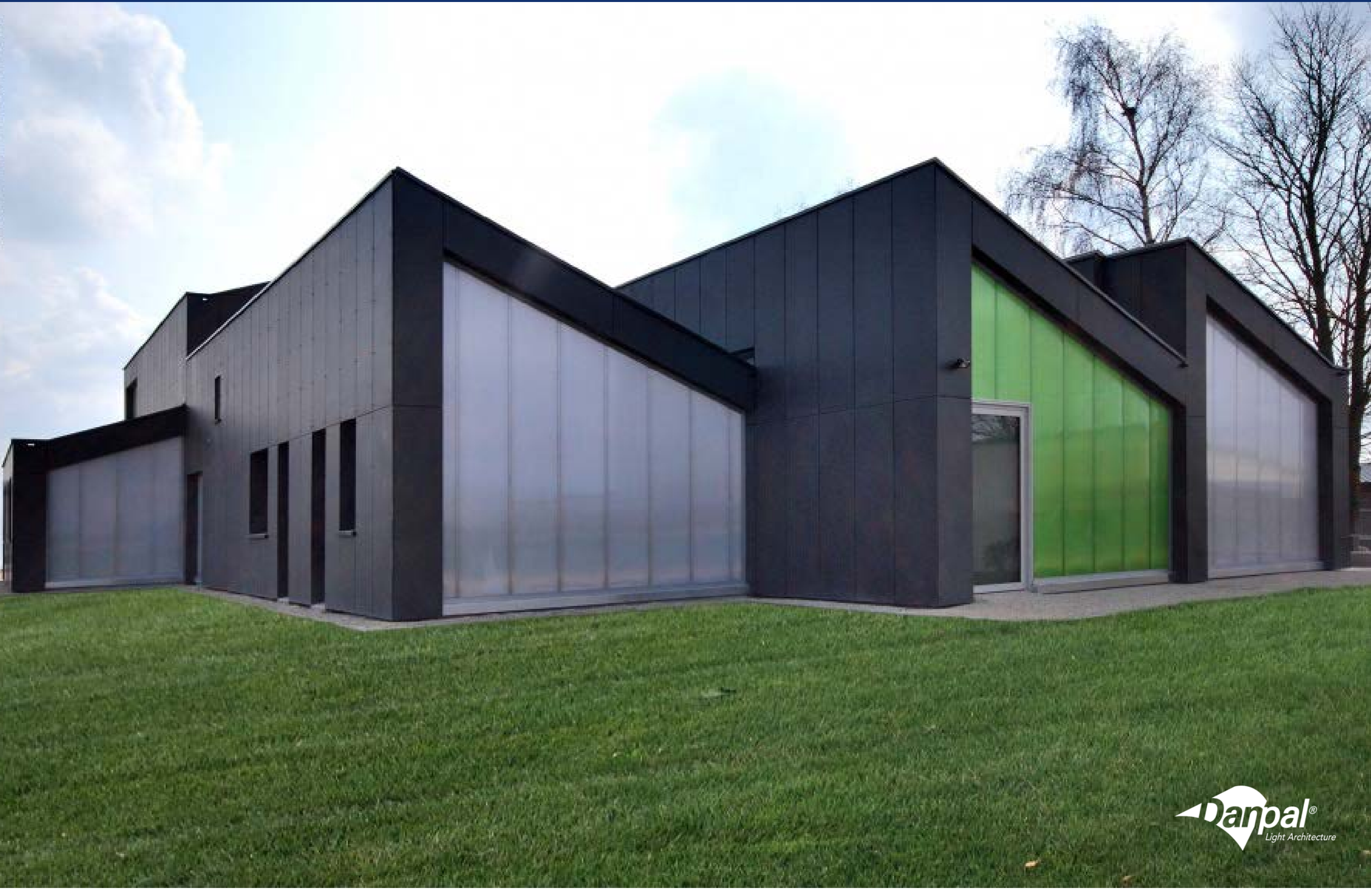
Industrial Building ,Atelier d'Architecture Sylvain GUITTET, France
